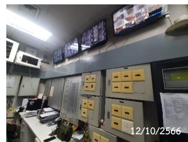
Graphic Annunciator Fire Alarm System
